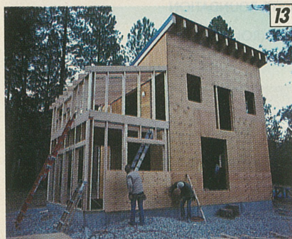
13 Once the main module is dried in, the greenhouse is framed, and sheathing starts to go on. You can build just the main cabin and add the greenhouse or other modules as you have time, need and money. The second floor above the greenhouse is also an optional module.
