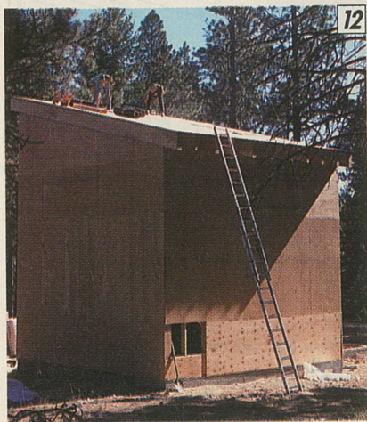
12 The house is dried in — wall and roof sheathing installed — as quickly as possible to beat the winter cold and allow comfortable working conditions inside to install drywall, flooring, etc.
