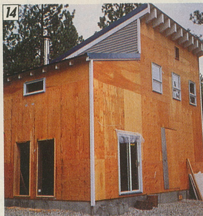
12 The house is dried in — wall and roof sheathing installed — as quickly as possible to beat the winter cold and allow comfortable working conditions inside to install drywall, flooring, etc.
